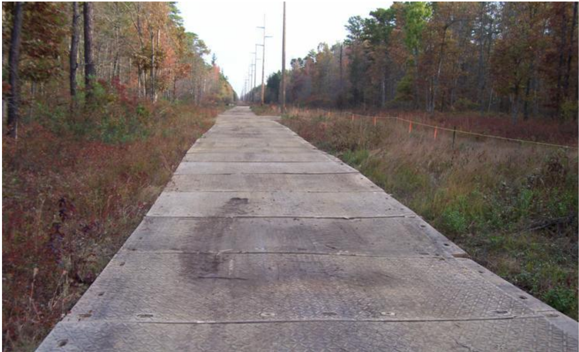
Figure 1. Matting Used for Transmission Line Construction (source: Black & Veatch)
