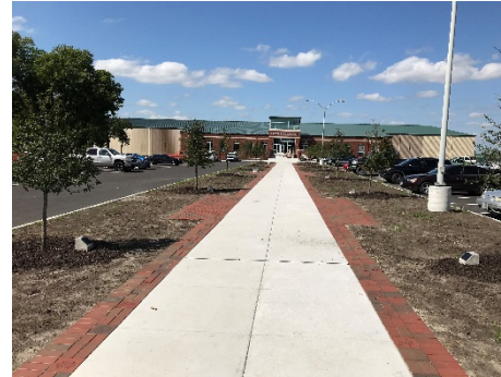
Progress – East Entrance
