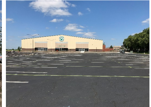
Progress – South Elevation
