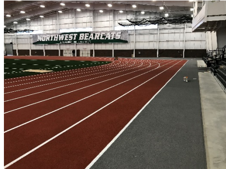
Progress – Activity Center
