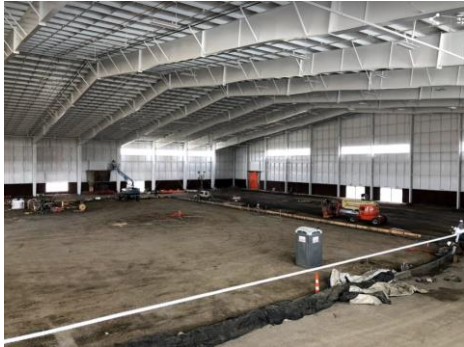
Progress – Overall Interior
