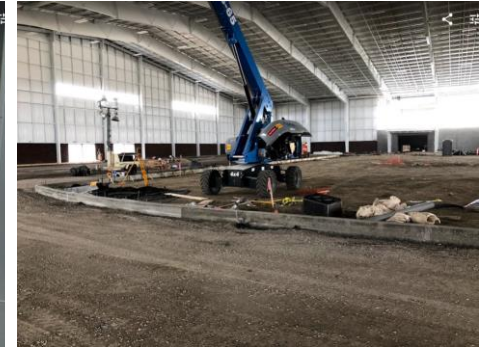
Progress – Interior Curb/Final Grading
