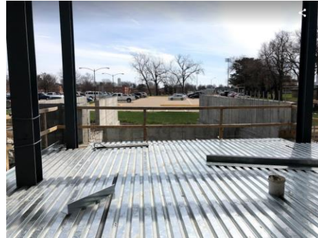
Progress – Upper Lobby East Elevation
