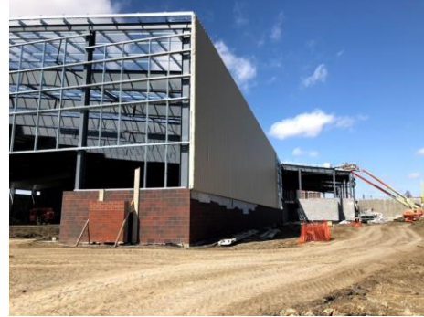
Progress - CMU/Support Bar
