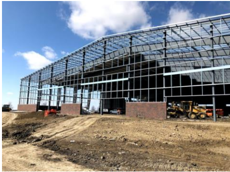
Progress – South Side
