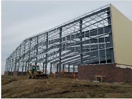
Progress – South Side
