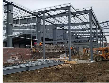
CMU/Support Bar Progress
