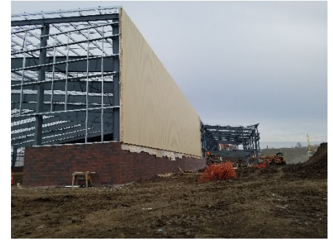
Wall Panel Progress
