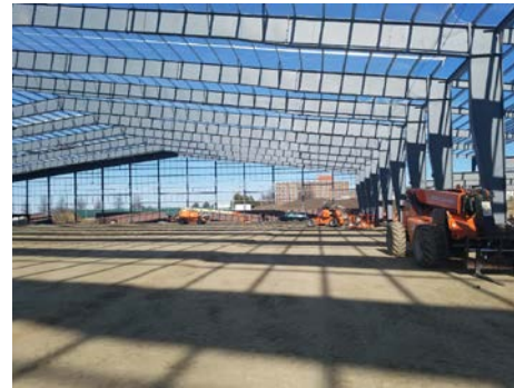
CMU progress – continues
