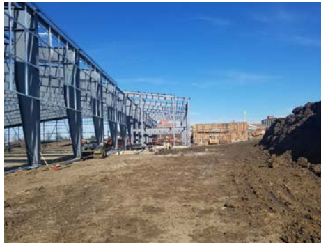
Support bar progress - continues
