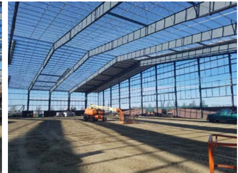
Main Bldg. roof started
