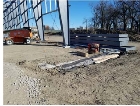
Interior/exterior drainage continues
