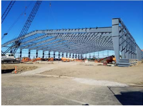
All main building columns set
