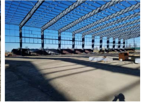
CMU continues along northwest
