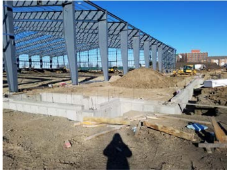
Support bar walls/footings continues
