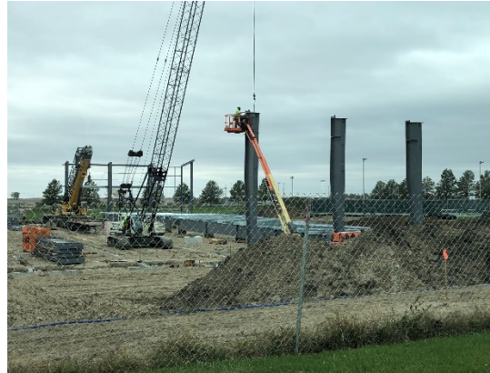
Erection of Steel Columns
