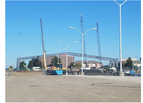
Erection of 1 st Bay Beams on North End
