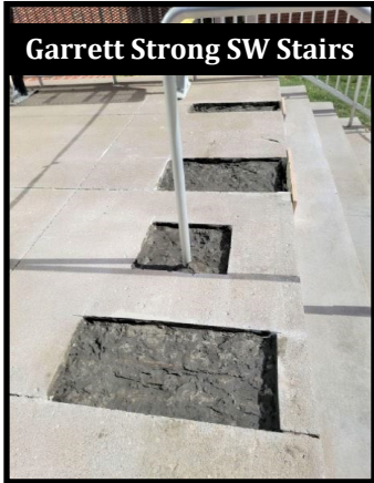
Concrete Patching
