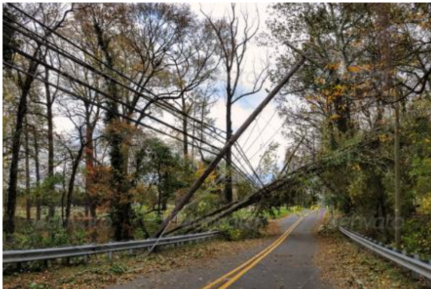
Figure 1.3 – Example of mechanical teardown (Photo by the Knoxville Utilities Board)
