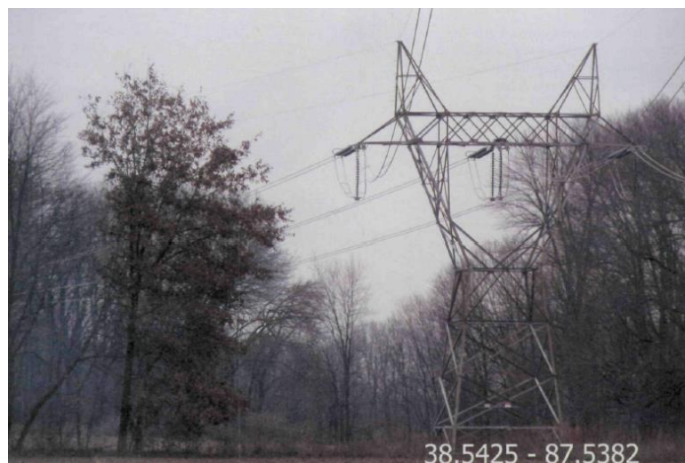
Figure 2.6 – A hazardous tree missed by AEP’s aerial survey but detected with LiDAR (Photo by AEP)
