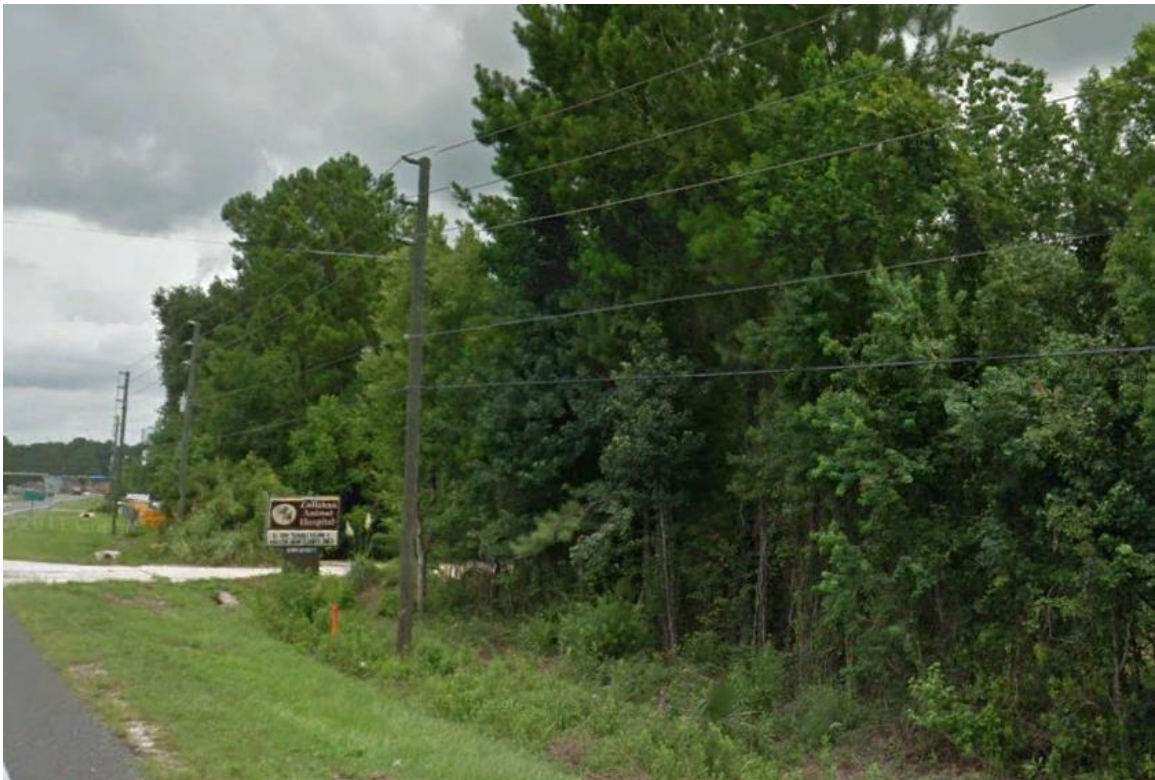
Figure 3.2 –Power lines found in the study area (GoogleEarth Pro).
